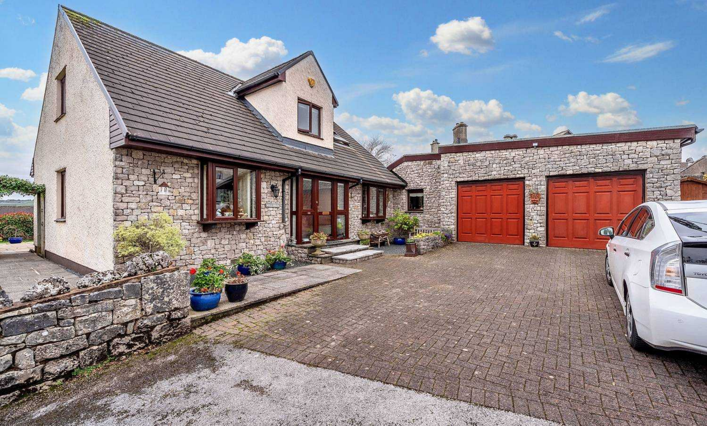
Well House Murley Moss Lane, Kendal £675,000
